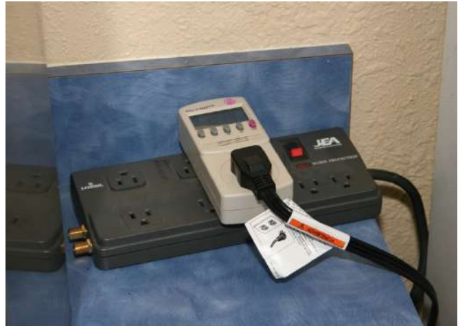
Using an extension cord for the refrigerator
