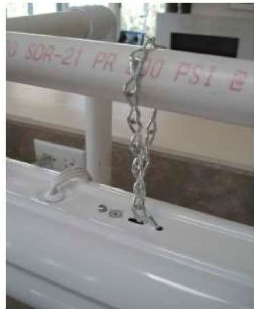
Figure 3 Detail of chain and "S" hook attachment
